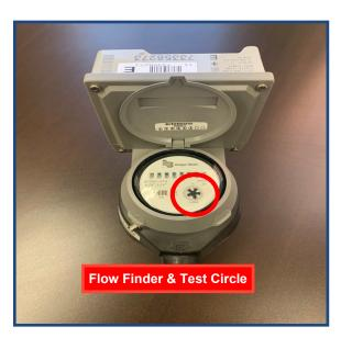
Above is a commonly used water meter in the Municipality of Strathroy-Caradoc. If you suspect a leak, you'll want to check the dial called the "Flow Finder & Test Circle" (shown in red circle). These are very sensitive and are useful in determining whether or not a plumbing leak exists. If water is not running in your home under a regular situation and the black wheel is still spinning, you may have a leak.
